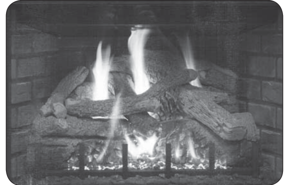
Fig. 51-2 Proper flame appearance
