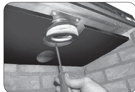
Fig. 54-4 Install plate and gaskets
