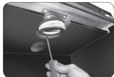
Fig. 50-4 Install plate and gaskets
