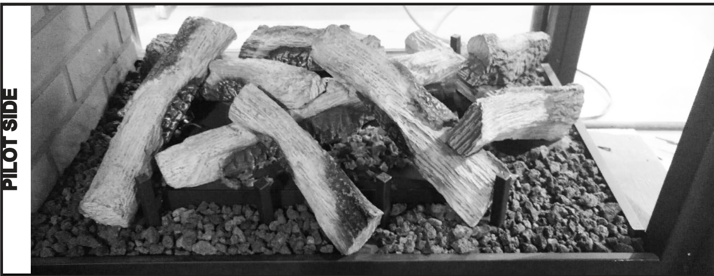
Figure 14. Log Set Installed
