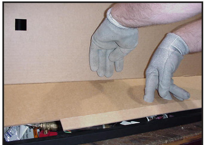
Figure 11.9 Opening Lower Access Panel
