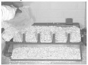
Figure 6 Placing Vermiculite
