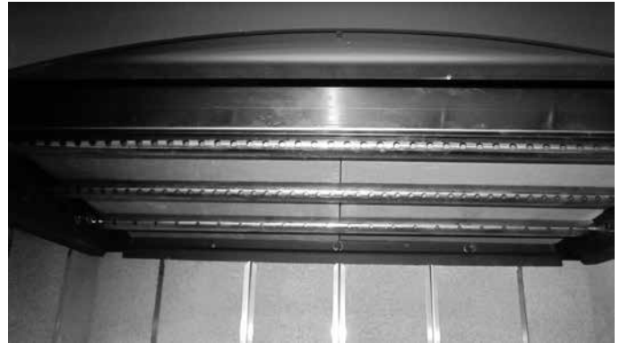
Figure 4.8 Reinstall Baffle Boards
