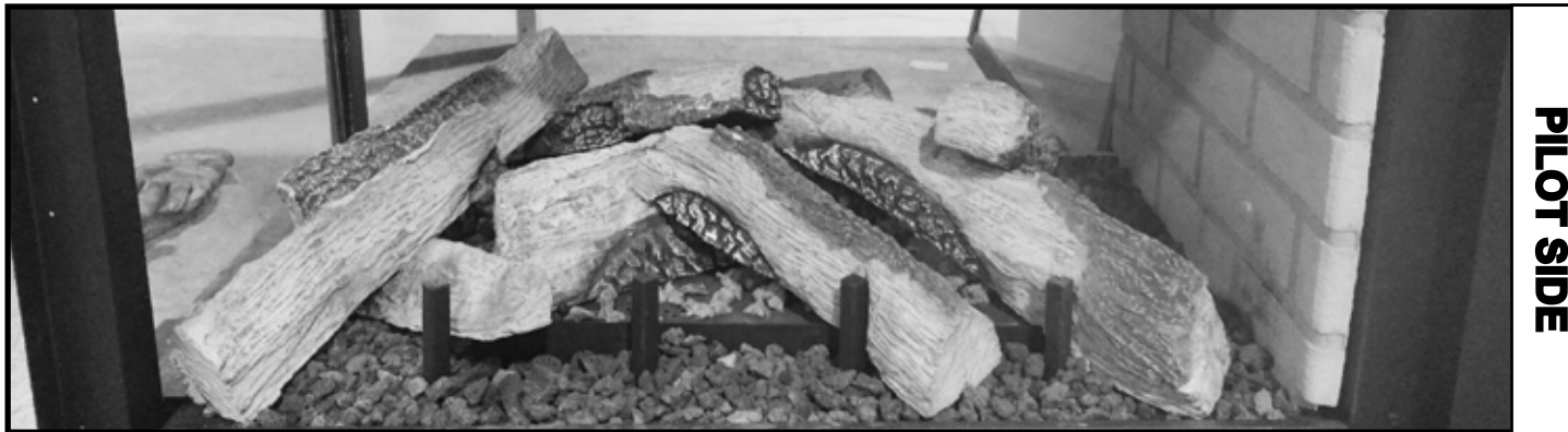
Figure 13. Log Set Installed
