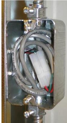
Figure 12 - Strain relief: If extension harnesses are used, connect them using a junction box, as shown. This will provide strain relief and ensure that the connection does not come apart.
