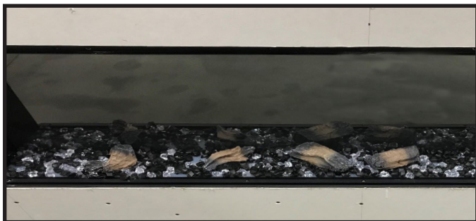
Figure 4.14 Media and Small Logs Installation
