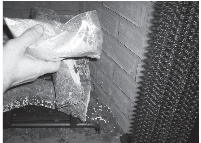
Figure 14.22 Placement of Vermiculite
