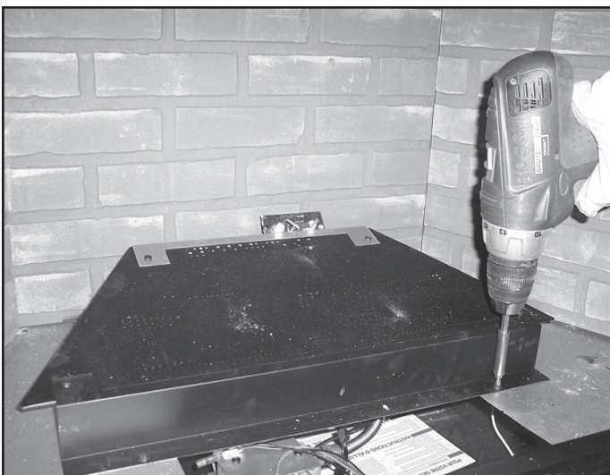
Figure 14.28 Remove Screws Attaching Front Burner Support
