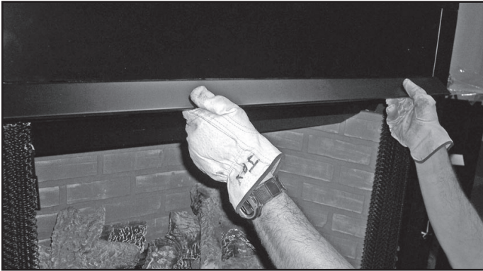
Figure 14.27 Installing the Hood
