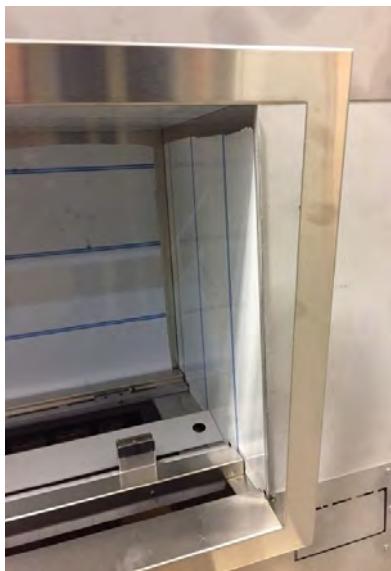
STEP 3: Hook Surround Frame onto Lower Edge of fireplace opening.
