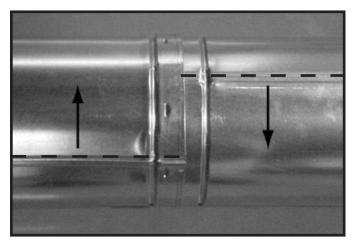
Figure 7.7 Rotate Seams for Disassembly
