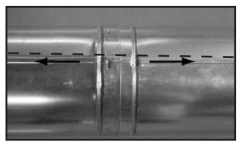
Figure 7.8 Align and Disassemble Vent Sections
