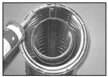
Figure 7.1 High Temperature Silicone Sealant
