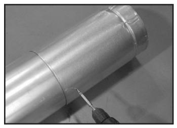
Figure 7.4 Screws into Slip Section
