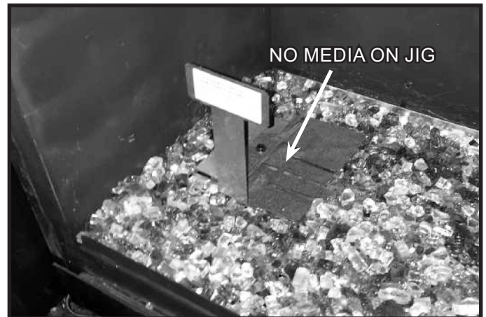
Figure 2. Media Placement Jig in Place
