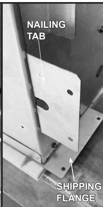
Figure 6.7 Nailing Tabs Installation Position
