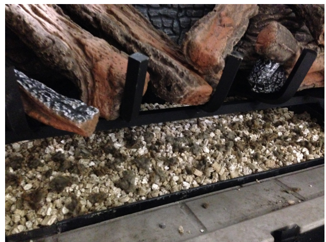
Figure 22 - Completed Installation of Vermiculite and Embers
