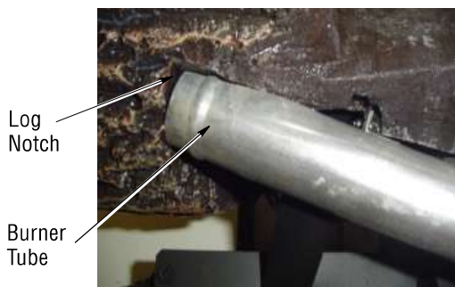
Figure 25A - Installing Back Left Log
