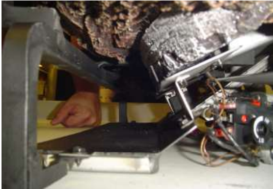
Figure 24C - Installing Right Front Log, Side View
