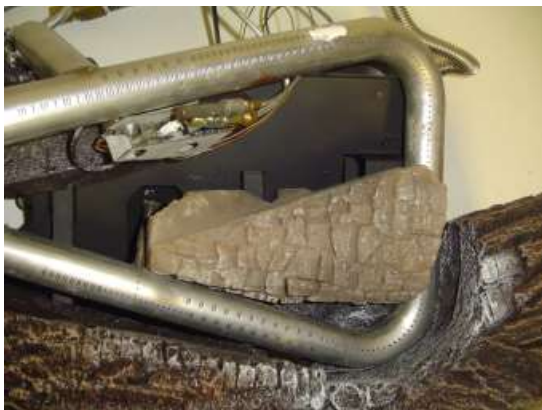
Figure 27A - Installing Charred Log Top View
