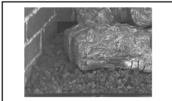
Figure 46 - Installing the volcanic stone
