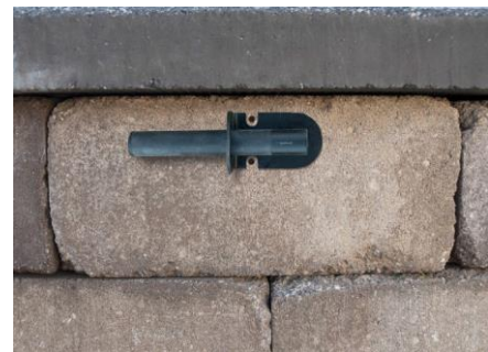
Figure 6.4 – Dry fit the bracket
