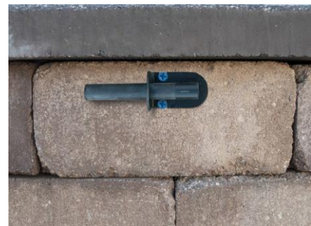
Figure 6.5 – Fasten down the bracket
