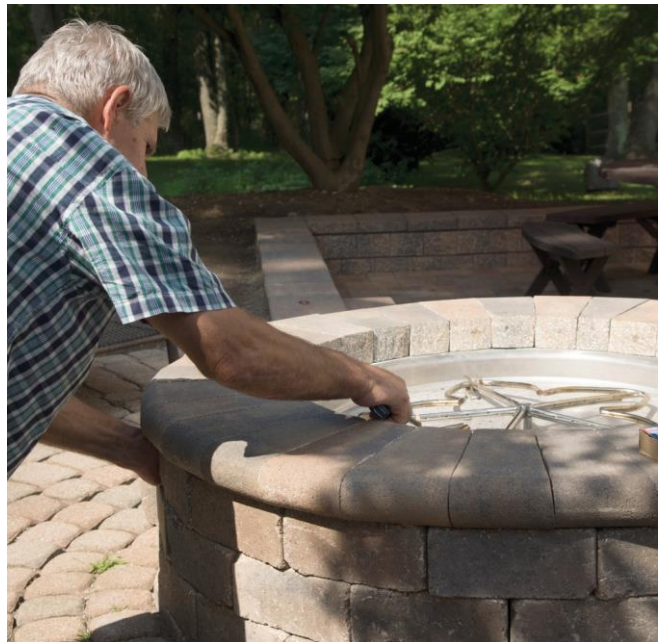
Figure 9.1 – Match-Lit test start-up
