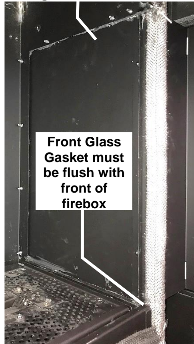
C Ensure Seal Gasket and Mill-Pac are sealed against the side of the firebox
