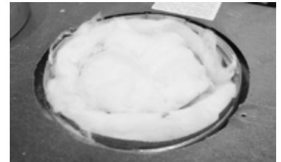
Step 3: Remove insulation from inside flue pipe.
