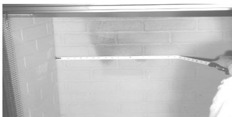
Figure 2.1 Measure Firebox
