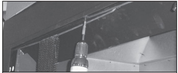
Figure 3.9 Removing the Screen Rods
