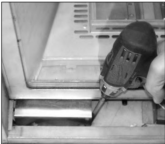
Power Vent Control Module Mounted inside fireplace.
