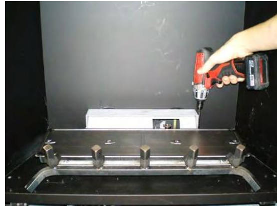
Step One: Remove Log Holder.
