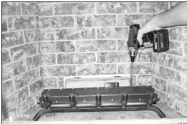
Step Four: Fix Side Liners in place using Liner Retainer Clips.
