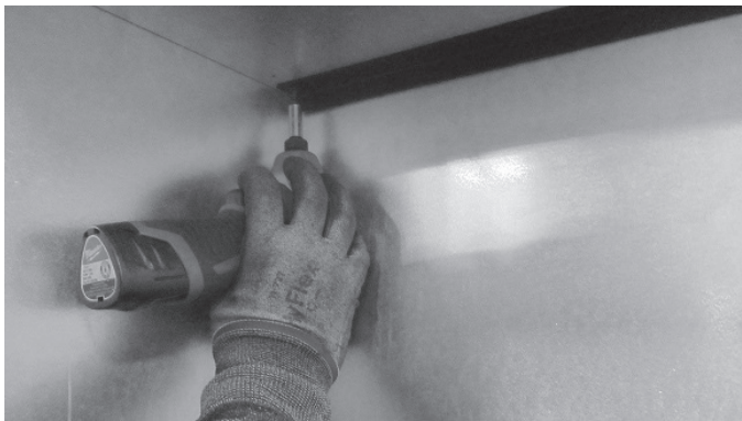
Figure 7.2 - Remove Rear Black Magic Glass Bracket
