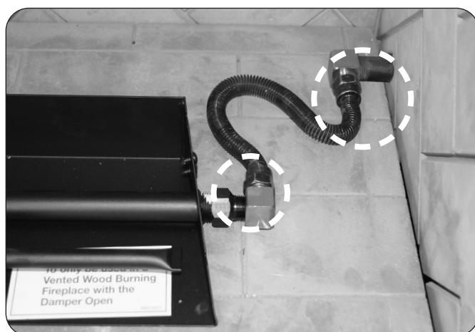
Fig. 9-3 Perform leak test
