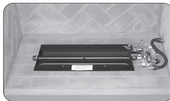
Fig. 18-2 Center burner in fireplace
