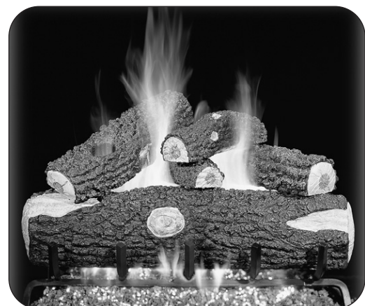
Fig. 58-3 Inspect burner flame appearance
