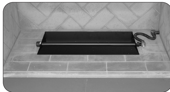
Fig. 10-2 Center burner in fireplace
