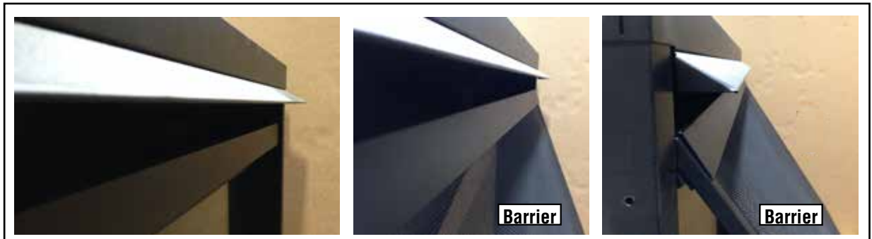
Figure 47A - Slide Barrier into Upper Trim Panel
