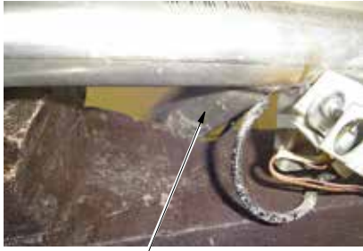
Vertical Portion of Burner Tube Figure 1B - Installing Back Left Log Rear View
