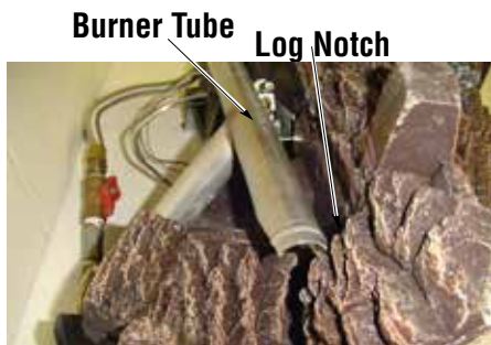
Figure 5A - Installing Middle Split Log Rear Top Side View
