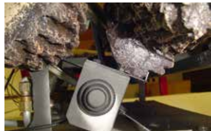
Figure 24A - Installing Front Left Log Side View
