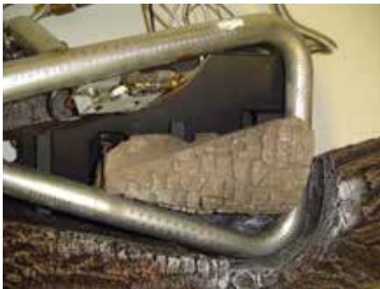
Figure 25A - Installing Charred Log Top View
