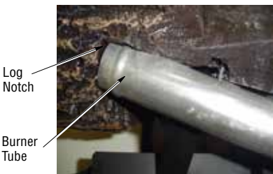
Figure 23A - Installing Back Left Log
