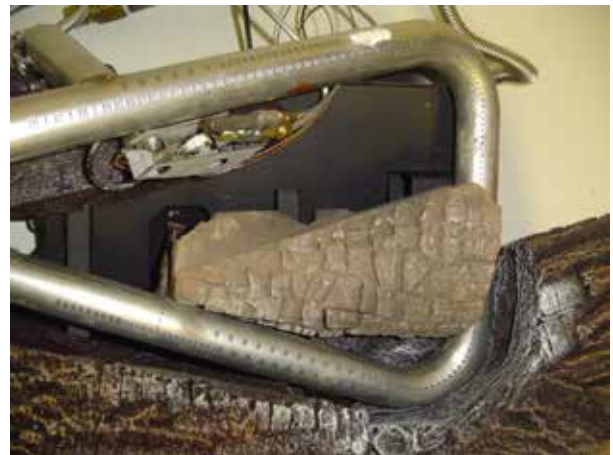
Figure 19A - Installing Charred Log Top View
