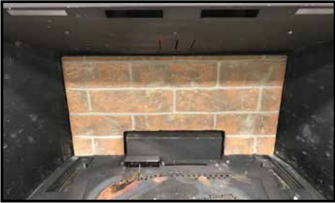
Figure 4 Back Refractory Installed
