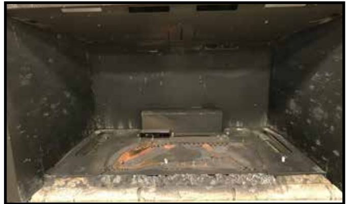
Figure 3 Base Refractory Installed
