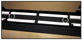
Figure 9 LED Retainer Bracket Removal
