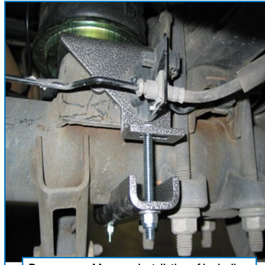
Passenger side rear. Installation of brake line.
