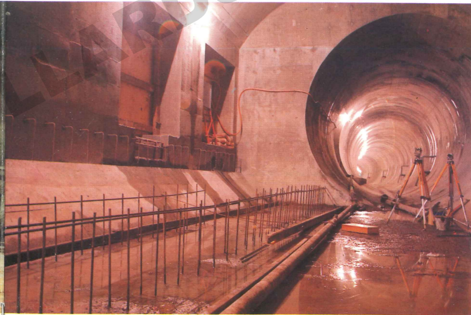
Flagstaff Station has required special construction methods because of ground conditions. Construction is proceeding to schedule. (Right) Making provision for escalators between platform and concourse areas. (Below left) Preparation for the installation of a pre-cast concrete platform, with a rail track to be laid on the right. (Below right) A platform tunnel viewed from one of the four running tunnels.
