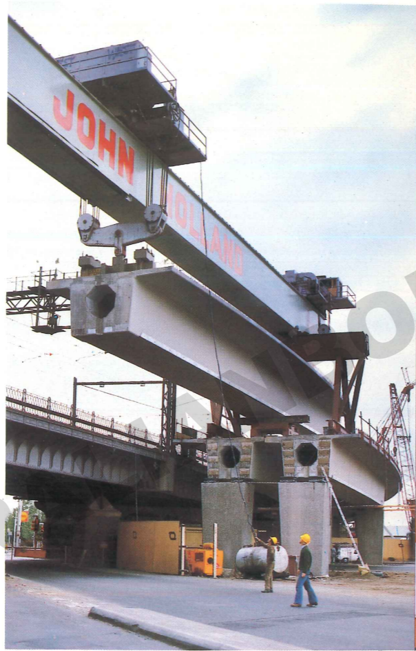
The provision of two additional elevated tracks between Spencer Street and Flinders Street Stations is a vital link in the MURLA project. The Overpass structure is 722 metres long and passes over five principal traffic routes. (Top) Overpass construction continues from beams already positioned. (Above) Overpass approaching completion. The existing viaduct is on the left with city buildings in the background. (Right) With an average length of 30 metres and weighing up to 290 tonnes, Overpass beams are positioned by launch girder winches with remote control.
