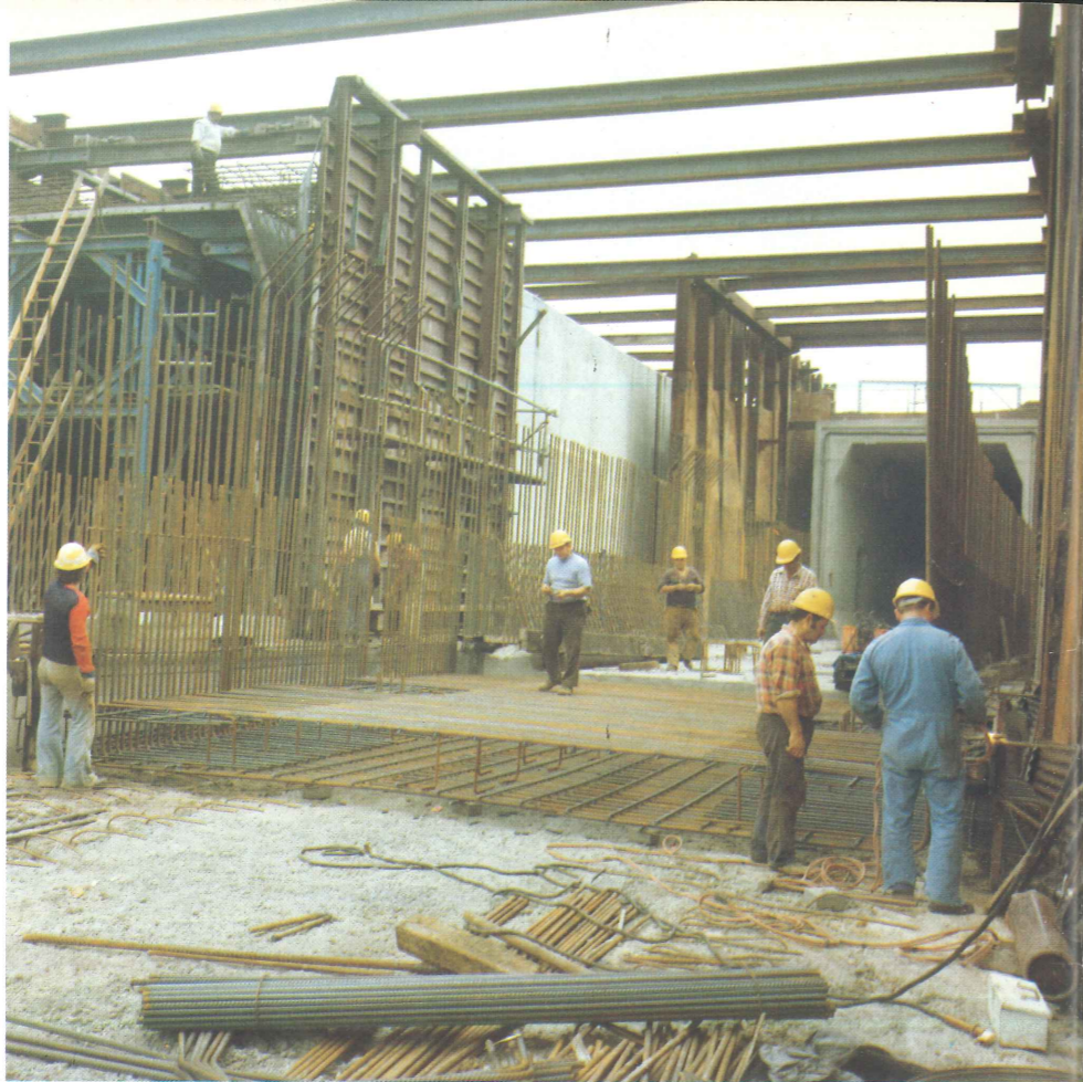
(Below) Platform tunnel for Parliament Station. (Right) Construction of box tunnels and ramps at north end of Platforms 9/10 Spencer Street Railway Station. (Lower left) "Y" junction of tunnels under Wellington Parade. (Lower right) Platform tunnel construction, Flagstaff Station.
