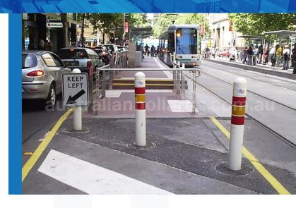
This is because of the bollards flexible design which allows it to 'give way' and 'absorb' the oncoming impact as it creates an obtuse angle that lifts the vehicle's front axle. This action in turn makes the passengers move back and away from the steering wheel and the dashboard, greatly reducing injuries and fatalities from occurring.
