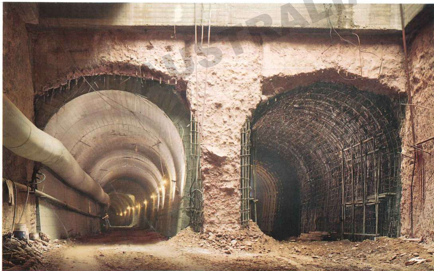
Excavation of the double track tunnel junction
