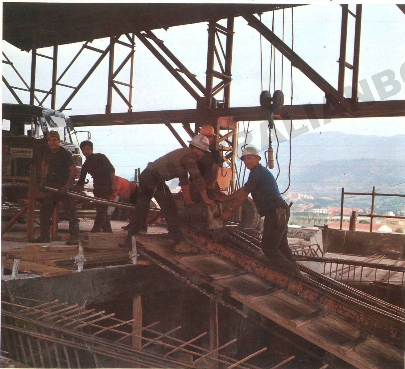
Positioning of the pre-stressing cables
