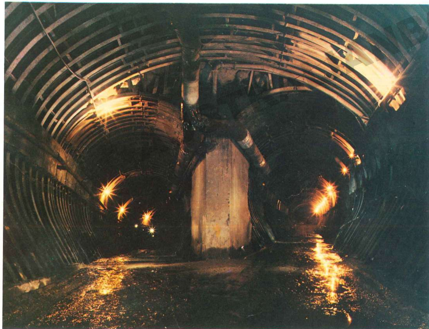
Later stages in the digging of the tunnel
