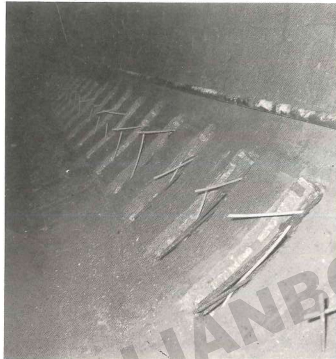
Details of recess for tensioning the cables
