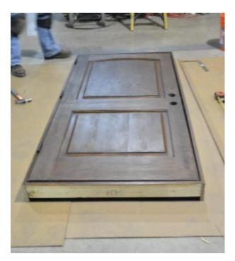
Step 8: Remove the weatherstripping from the legs of the door frame. Please pull gently on one end (either the top or bottom) to be careful not to tear the weatherstripping. \*Place to the side for later reinstallation.
