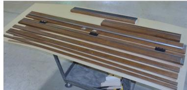
Step 3: To begin the assembly of this door unit: Lay down something to protect the door and/or finish on a flat, level surface. This can be any cardboard pieces or packing material from the door crate. Place the header and two legs of the door frame with the thicker side down on the floor.
