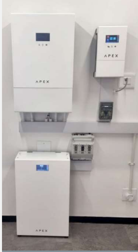
Figure 3. B12K Typical Installation, Connected With A Fuse Disconnecter
