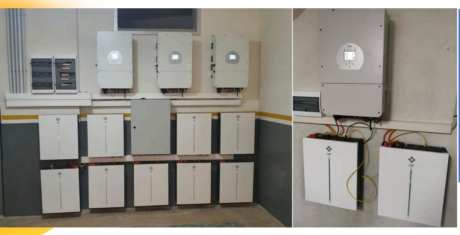
For this kind of installation scenario, with busbar, installer can use the power cable which a part of CA03 to connect battery to busbar, but need prepare an additional standard straight CAT5 ethernet patch cables for the communication between batter packs.
