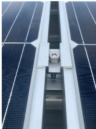
Figure 2 ASCENT Kliplok mounting using the mid clamp to clamp 2 panels and the end clamp to clamp the panels at the end of a string
