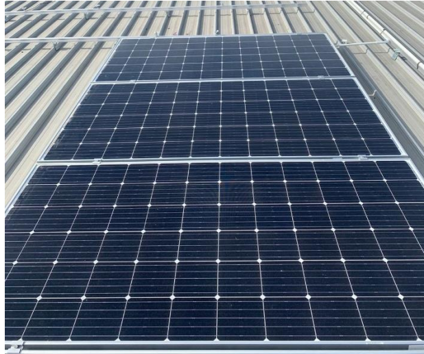
Figure 1 ASCENT mounting structure for Kliplok roofing sheets
