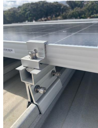
Figure 2 ASCENT Kliplok mounting using the mid clamp to clamp 2 panels and the end clamp to clamp the panels at the end of a string
