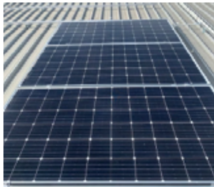
Figure 1 ASCENT mounting structure for Kliplok roofing sheets
