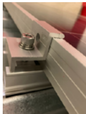
Figure 2 ASCENT IBR mounting using the mid clamp to clamp 2 panels and the end clamp to clamp the panels at the end of a string
