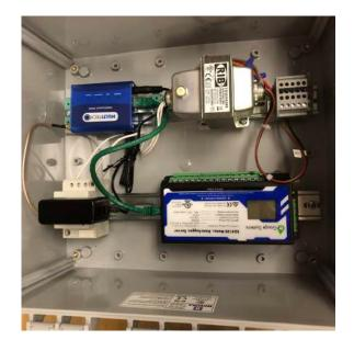
10) Connect the power adapter for the cell router to the 120VAC receptacle and the Ethernet cable to the eGauge
