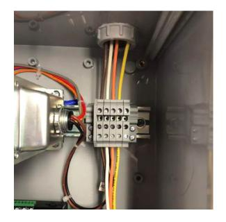
12) Wire the power distribution block to a breaker or fuse block of the distribution panel being measured.
