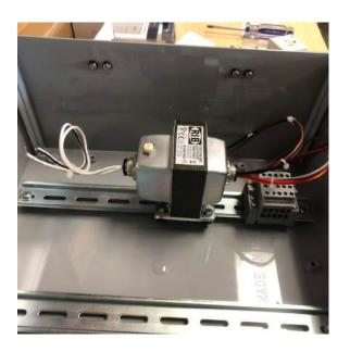
4) Connect the 50VA Potential Transformer to the same DIN rail as the terminal block. Orient the primary side (colored wires) toward the terminal block. The black wire on the primary side of the transformer is the neutral line.
