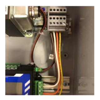
11) Cut lengths (about 7" long) from each of the 15' colored cable, strip about 1/4" from each end, and use each to connect the eGauge voltage block to the power distribution block.
