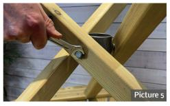
**4.** Once the legs are in place, screw and attached them into the tabletop using the pre-drilled holes. When screwed in, tighten up each bolt connecting to the circular hinge (see pictures 4 and 5).
