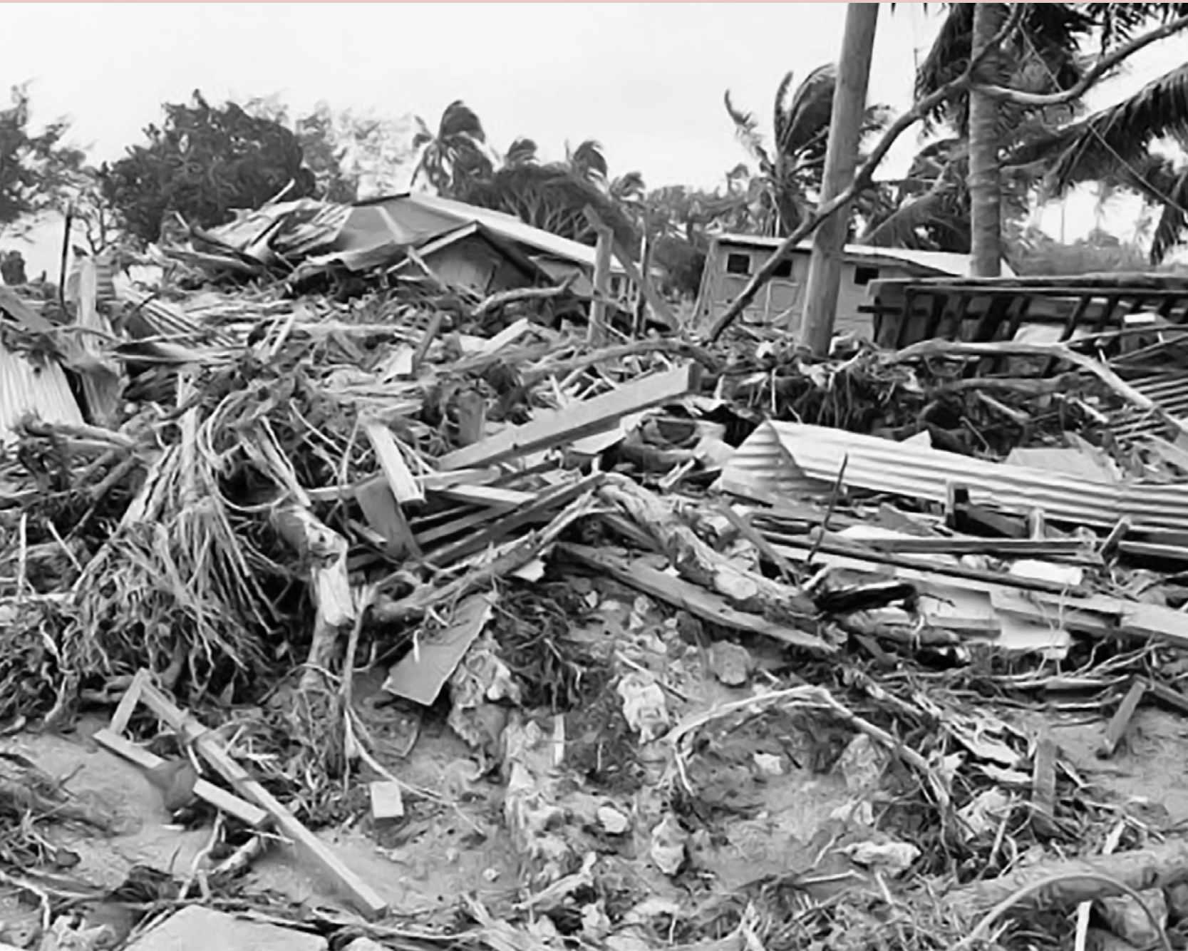
February 2018 — Path of destruction left behind Cyclone Gita in The Kingdom of Tonga.
