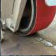
Weld seam and heavy sheets grinding
