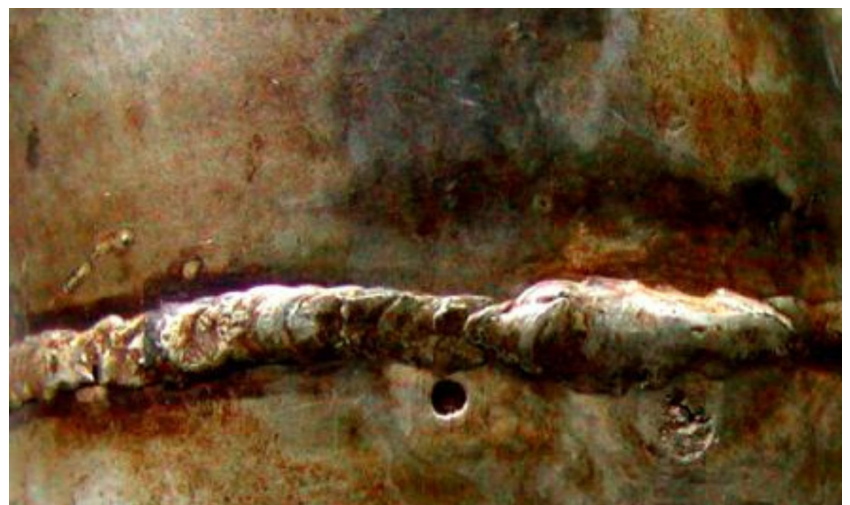
Example of pit corrosion caused by the presence of embedded iron
