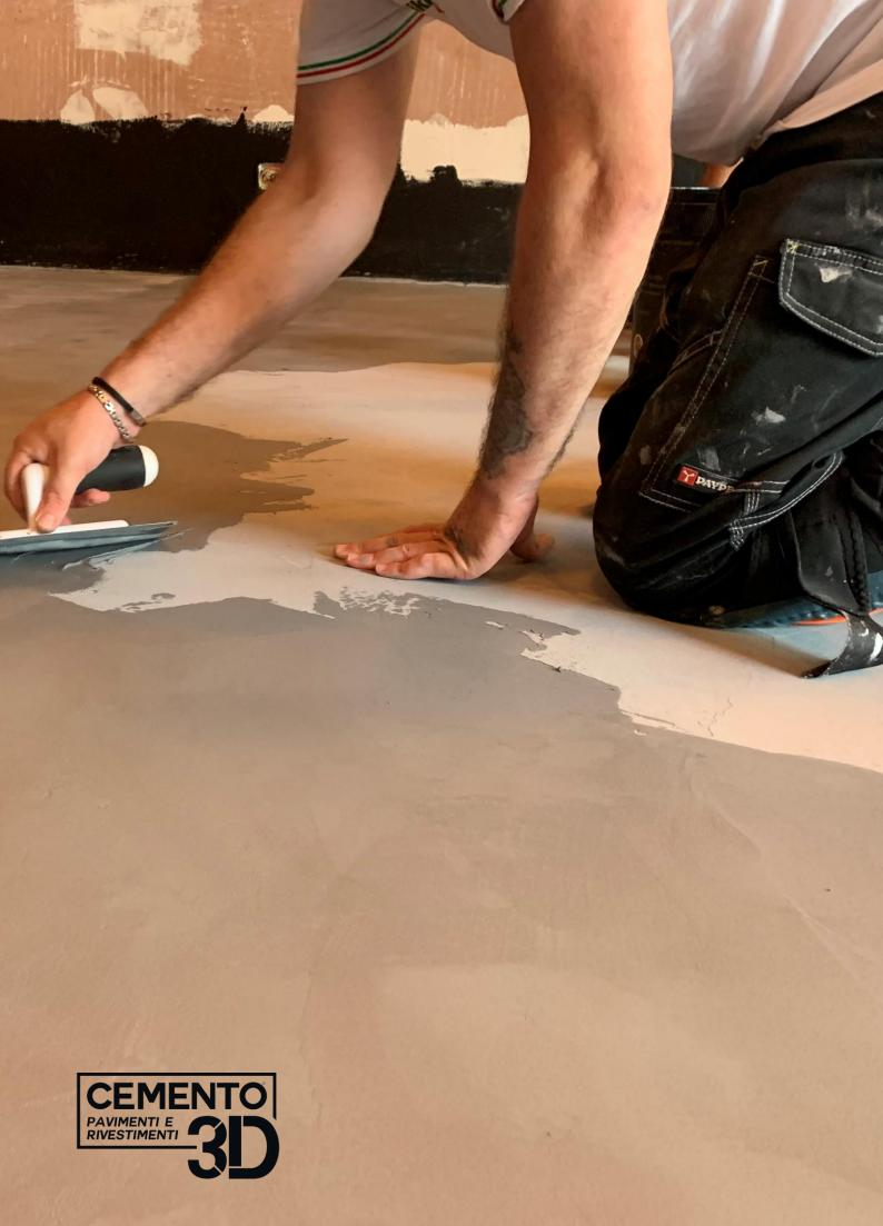
Cemento 3D is a new generation structured nanocement, premixed in powder form composed of selected quartz sands and marble powders, minerals, nano resins and special additives.
